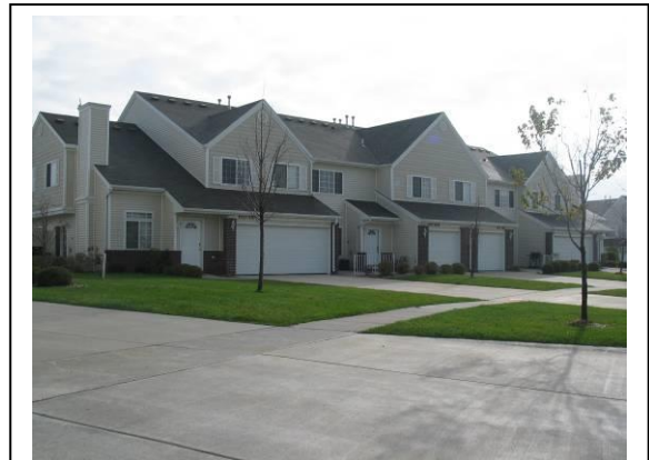
Example of Single-Family Attached
