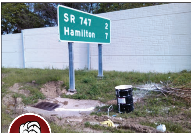
Fig. 2-11. Materials should be stored in designated areas and not with direct discharge to unprotected inlets.
