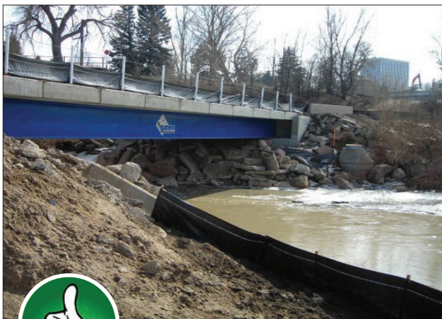
Fig. 5-3. Temporary bridge with good sediment controls on bridge and embankments.
