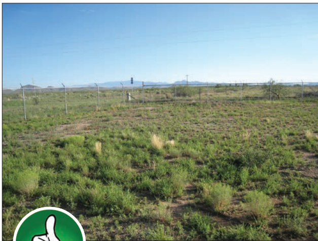
Fig. 1-11. Final stabilization is reached typically at 70 percent uniform cover. That percentage should be applied to the percent cover of pre-existing conditions.
