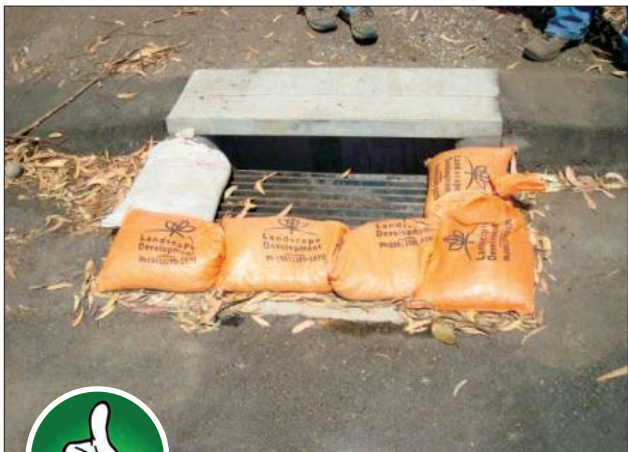
Fig. 5-9. Use of gravel bags is among the most common approaches to inlet protection.
