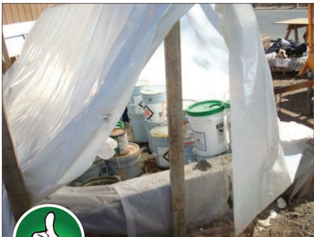
Fig. 2-3. Paints should ideally be stored inside. When this is not possible, a tarp or cover is the next best option.
