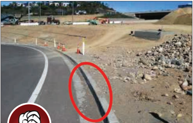
Fig. 3-3. Notice the sediment within the gutter caused by lack of perimeter controls. Source: Nevada DOT
