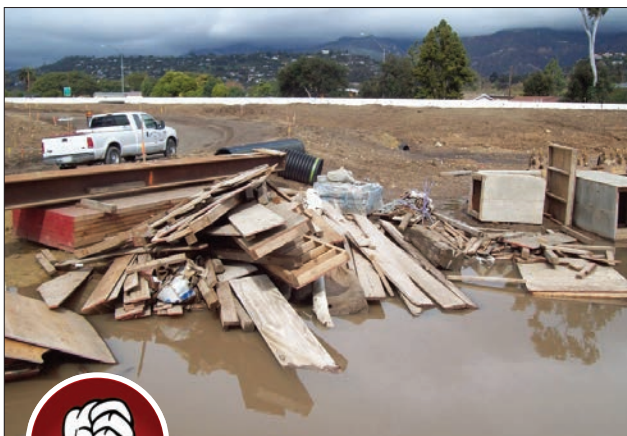
Fig. 2-7. Waste and debris permitted to come into contact with large amounts of drainage represent a significantly greater environmental risk.
