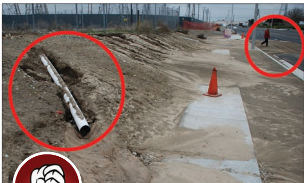
Fig. 5-29. Failure to effectively stabilize this pipe at the outlet, among other failures, leads to a larger slope erosion problem and sediment discharge into the gutter. Source: RBF Consulting
