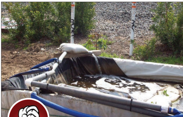
Fig. 3-16. Remember to stop dewatering when reaching capacity (filtering bags at right nearly submerged) or when bags fail to filter sediment.
