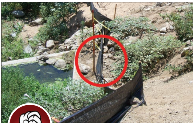
Fig. 3-5. Too much dirt can cause the silt fence to tip over or break.
