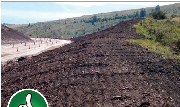
Fig. 4-1. Track walking is among the most common techniques used to roughen a slope. Grooves should be created along the slope contour line.
