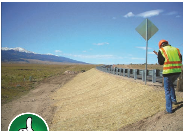
Fig. 4-14. This is an excellent installation of soil retention blankets. The blanket is entrenched at the top and bottom of the slope.
