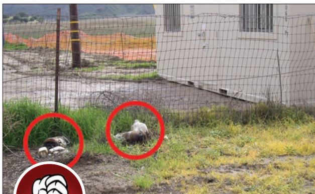
Fig. 2-16. Illegal dumping often occurs at the perimeter of the site, where access is hardest to control. Source: RBF Consulting
