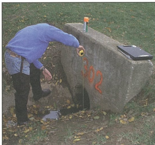
Figure 27: Measuring Outfall Diameter
