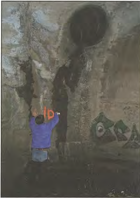
Figure 24: Labeling an outfall (a variety of outfall naming conventions can be used)
