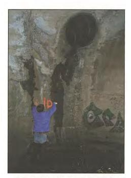
Figure 24: Labeling an outfall (a variety of outfall naming conventions can be used)
