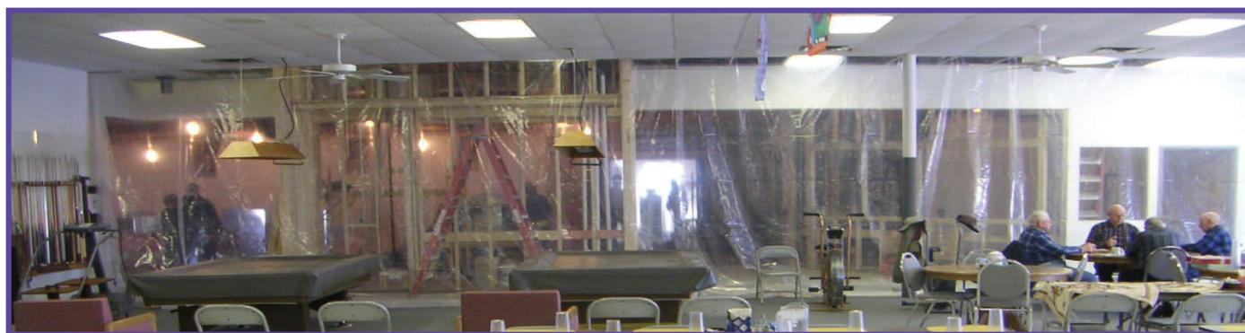
Interior progress of Grand Generation Center on January 23, 2007
