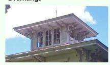
Properly sized and installed roof overhangs can most effectively shade south-facing windows from summer heat. If oriented properly, overhangs will allow sunlight in through the windows during winter, providing more warmth to a house.
