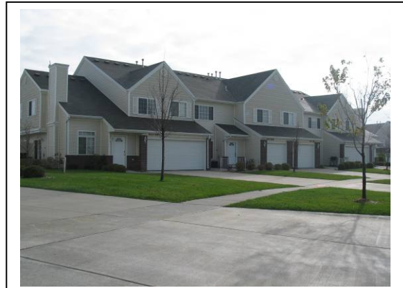
Example of Single-Family Attached
