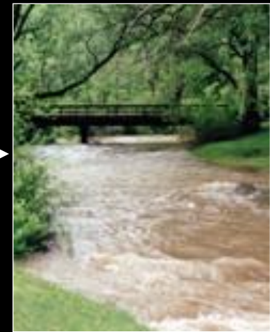
Sedimentation and flooding during rain event
