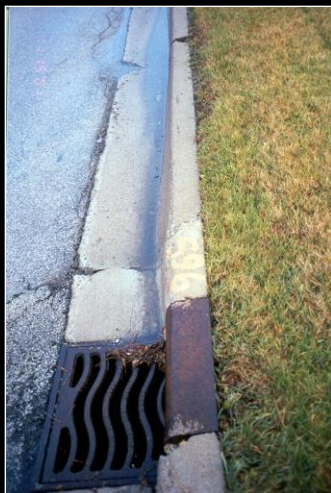
Typical roadside catch basin
