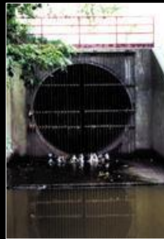
Storm drain outfall
