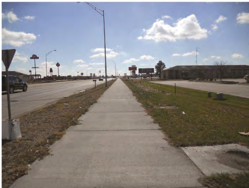
Existing Conditions along Plum Creek Parkway
