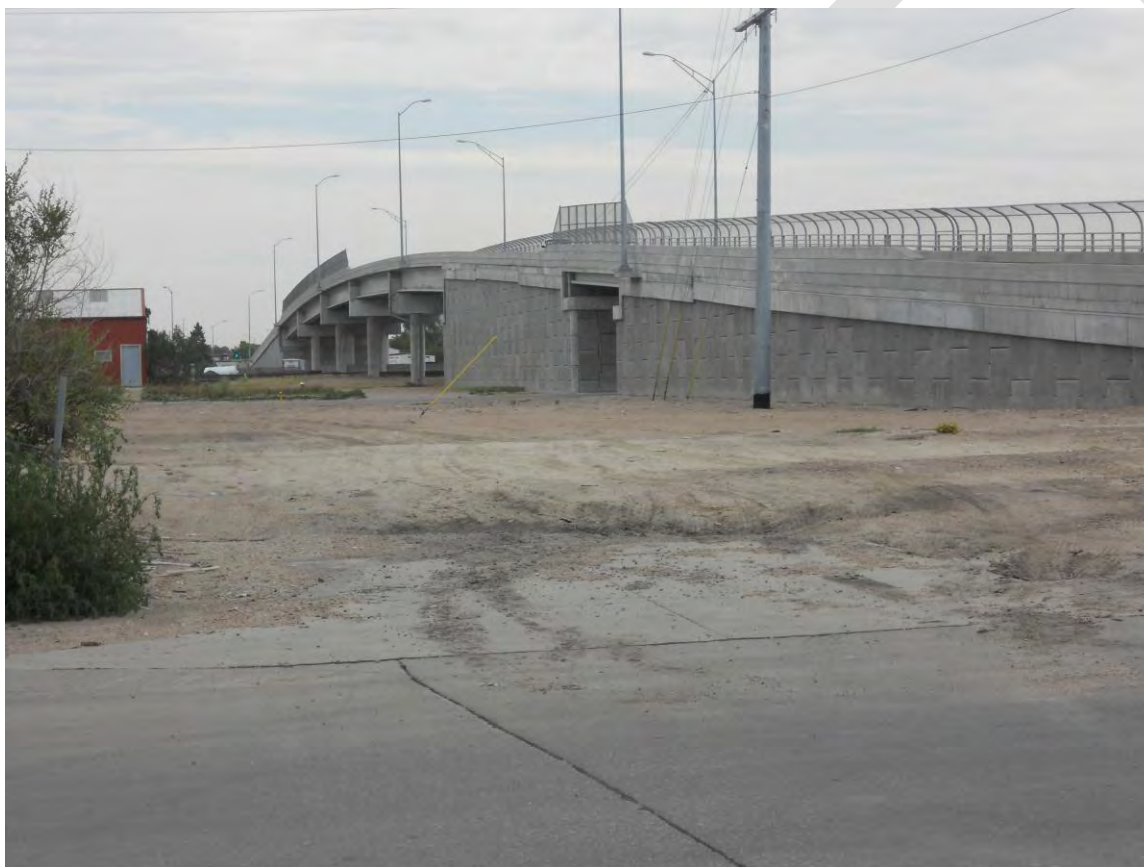
U.S. 238 and Jackson Street Bridge
